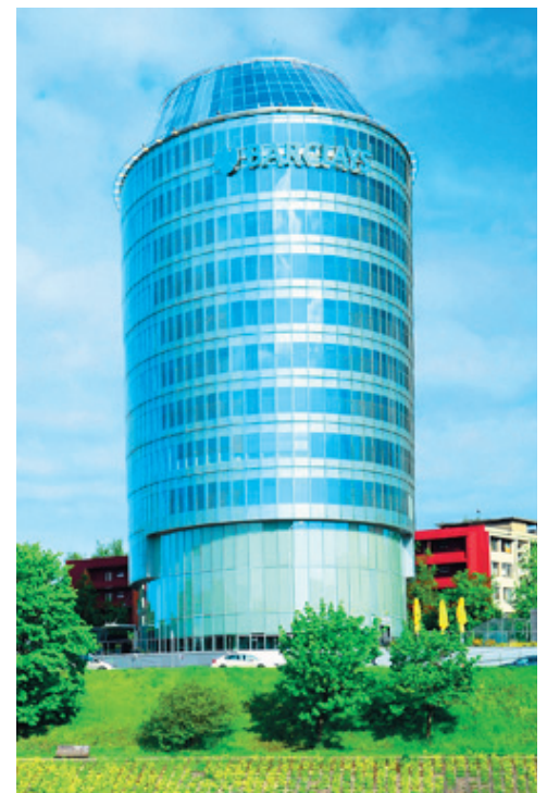
A metal building.
