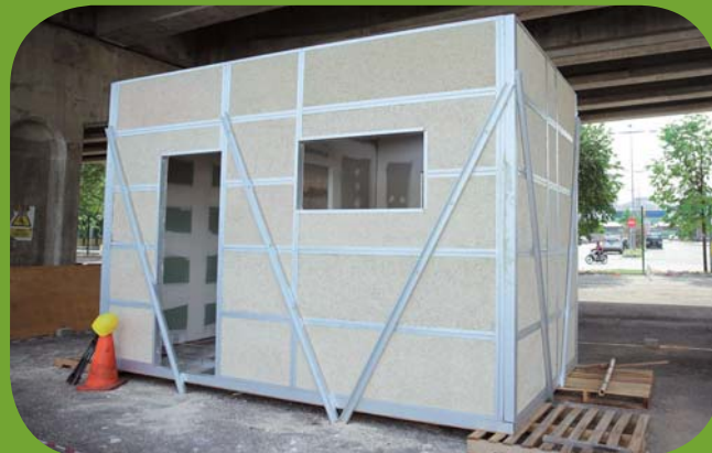
Work in progress of the tiny home back in October last year.
