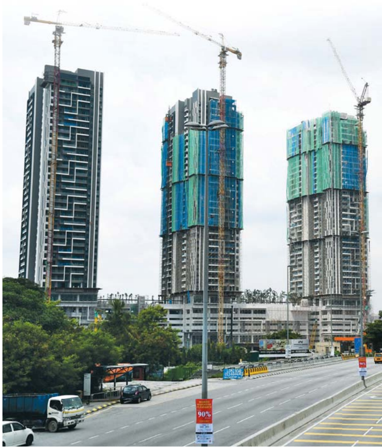
The construction of Citizen 2 by Binastra Land along Old Klang Road
