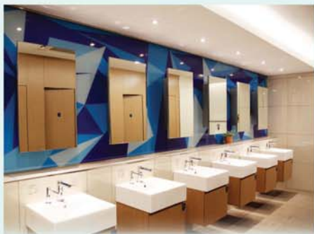
New toilets with auto-sensor taps, soap dispenser and wash closet flush system.
