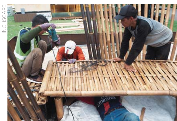
Bamboo was the main material used for the garden.
