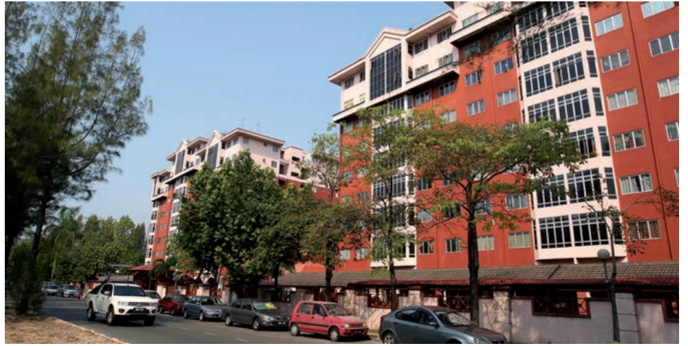
Permai Villa commands the highest growth in capital values due to its strategic location to two upcoming LRT stations in Taman Puchong Perdana.
