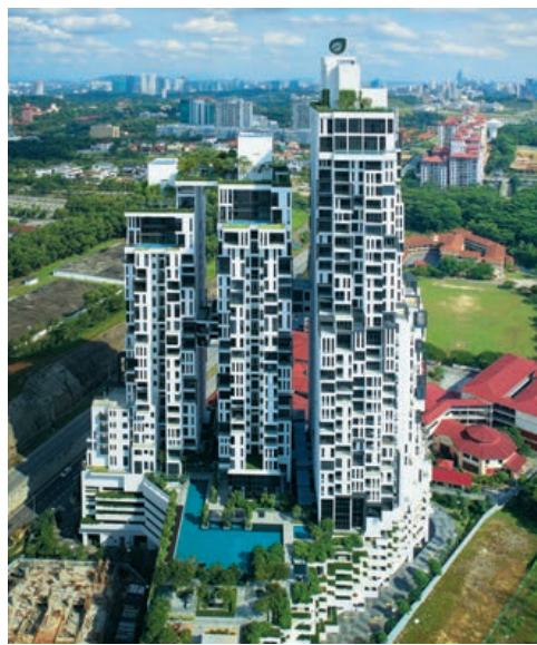
An aerial shot of the completed Icon Residence Mont'Kiara. Photo by Mah Sing
