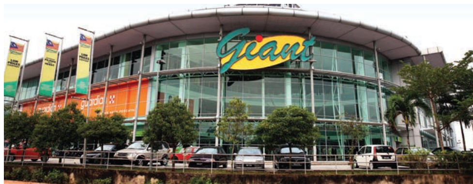
Giant Kinrara in BK5 is close to a future LRT station.
