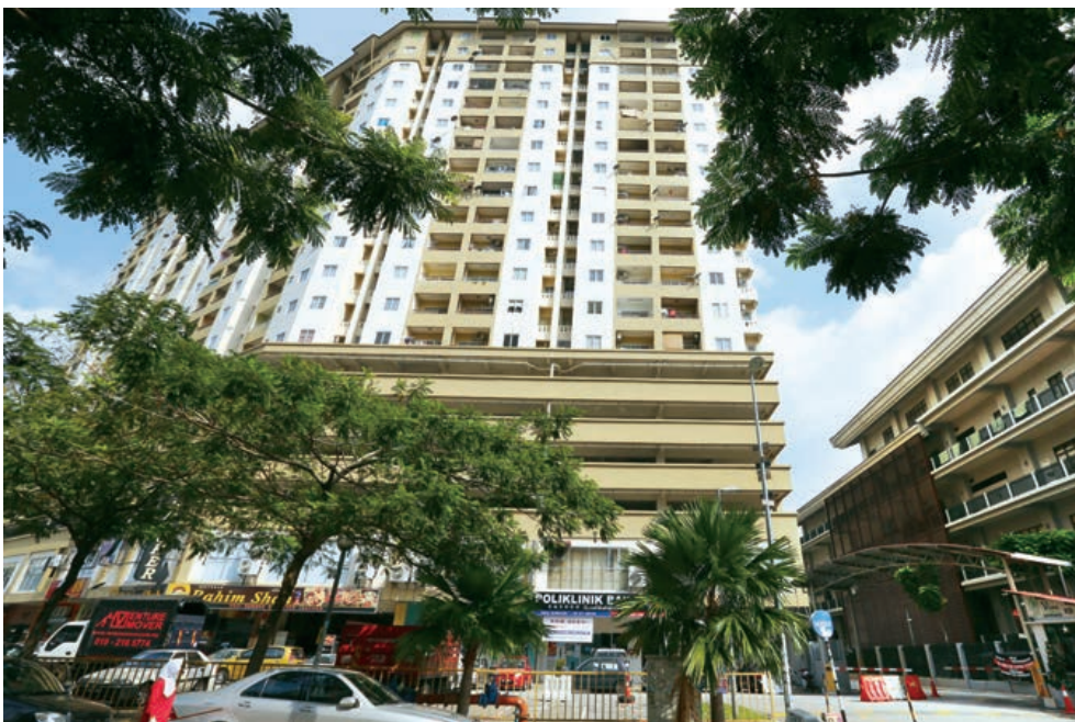
Vista Mutiara is one of the most expensive high-rise developments in Kepong.
