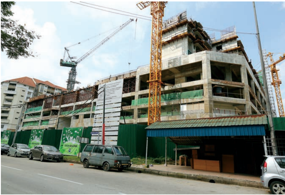
Fortune Perdana Lakeside is under construction.
