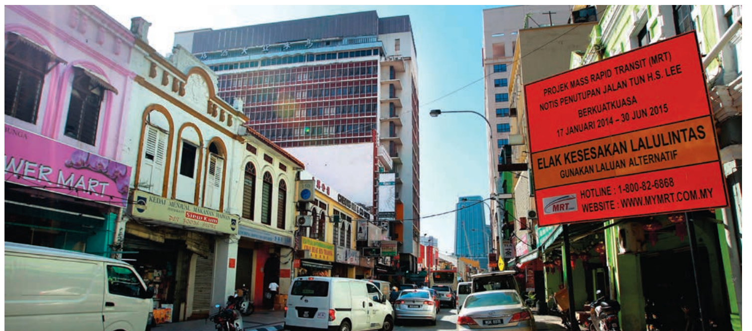
Road alignment along Jalan Tun H S Lee due to the MRT station construction. Photo by Shahrin Yahya/The Edge Property
