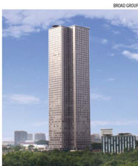
The Mini Sky City in Hunan, China was completed in 19 days using modular construction methods.
