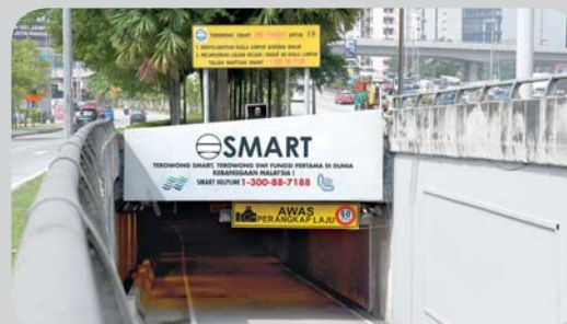
Stormwater Management and Road Tunnel (SMART Tunnel), Kuala Lumpur
