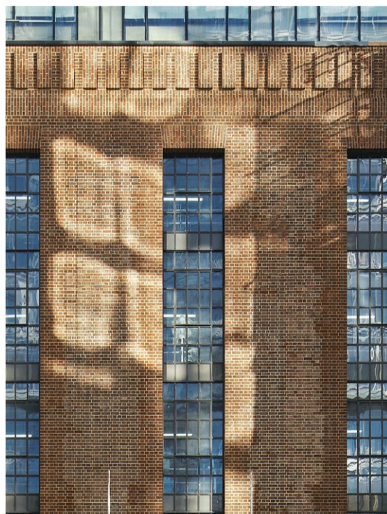
About six million bricks were used to construct the old power station back in the 1930s.
